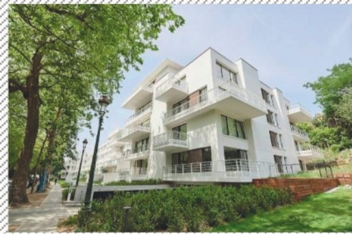
EAGLESTONE // AXENT ARCHITECTS
