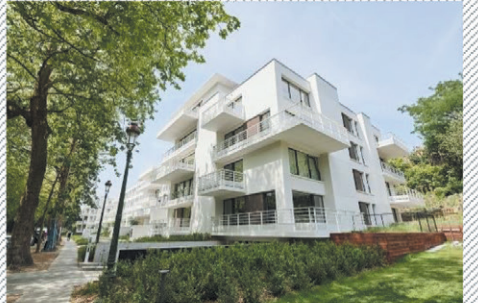
EAGLESTONE // AXENT ARCHITECTS
