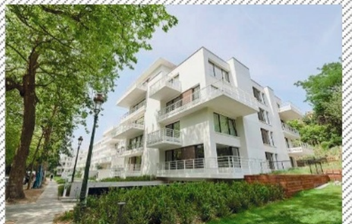
EAGLESTONE // AXENT ARCHITECTS
