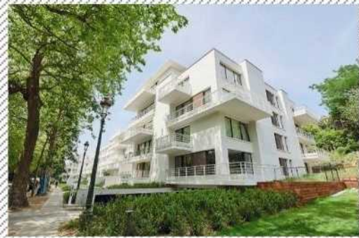
EAGLESTONE // AXENT ARCHITECTS
