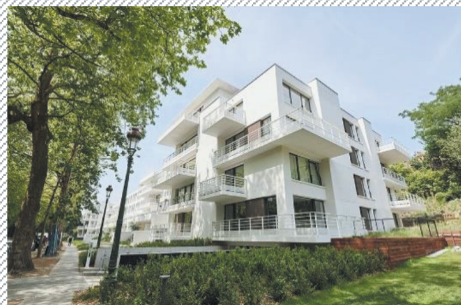
EAGLESTONE // AXENT ARCHITECTS
